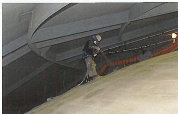
Figure 6. Application of new PU foam.
