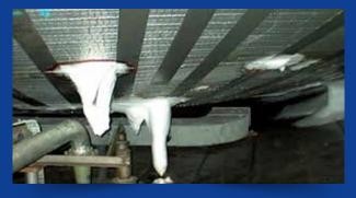
MOSS LNG insulation is prone to a variety of defects typically showing after time and can be observed as extended de-lamination of vapour barrier and spray shielding, extensive and frequent surface cracking as well as complete through thickness cracking.
