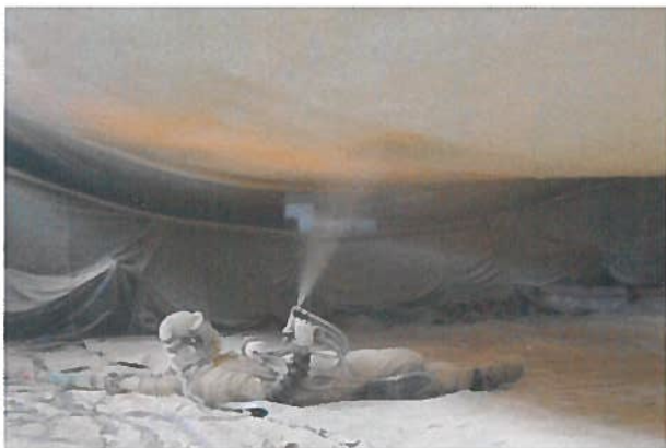
Figure 1. Spray foam installation.
